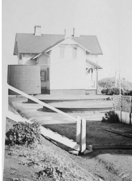
1894 photo of in-ground cisterns. Above-ground cistern by west side of double keeper's dwelling is at far left. Photo by Herbert Bamber. Courtesy of the National Archives.
